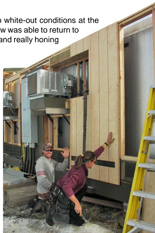
Dan Lindberg and Annalisa Gross working construction at Toolik.
